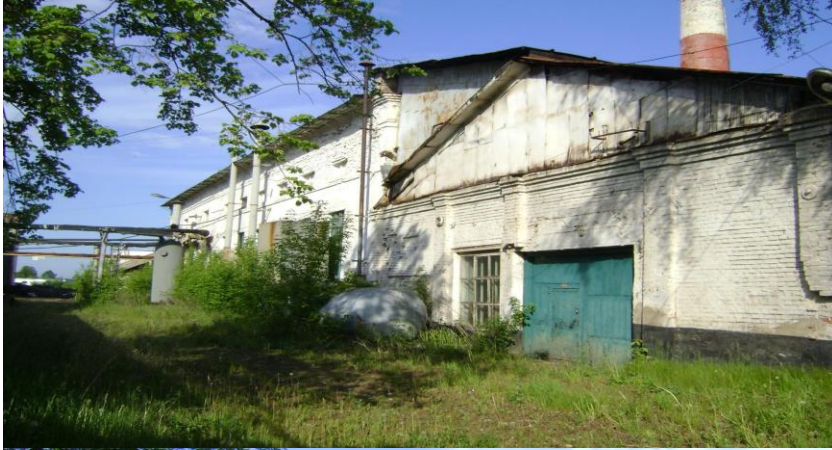
Compressor station with main facility and electrical laboratory, measuring and recording apparatus
