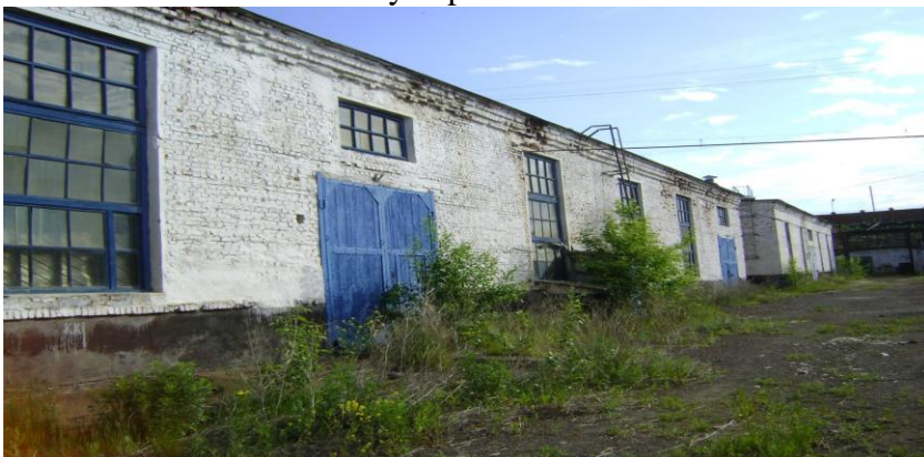
Prefabrication and assembly department and storeroom N 2
